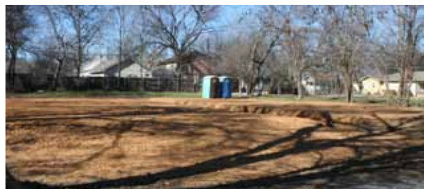
Two lots have been cleared for construction of the first two new homes.
