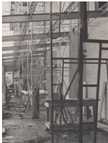
Construction of the Education Wing
